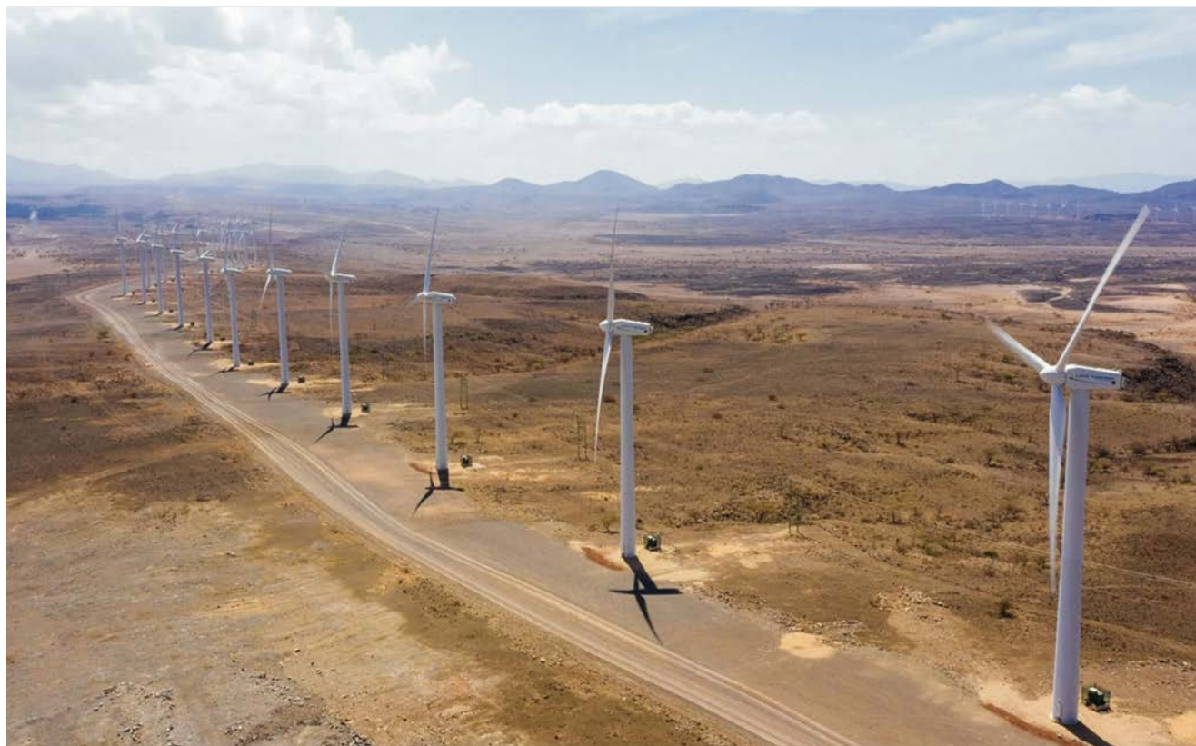
Kenya's Lake Turkana Wind Power project comprises 365 850KW wind turbines and a high-voltage substation (LAKE TURKANA WIND POWER)
